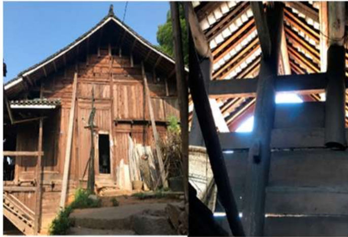
Figure 14: Wooden exterior wall and Double-tile roof (Source: Sustainability, 2021)
